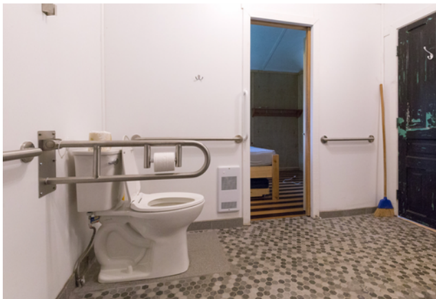
The washroom is equipped with grab bars
