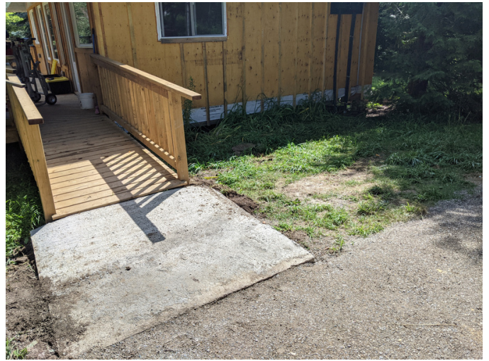
Dave's cottage ramp with hand railing
