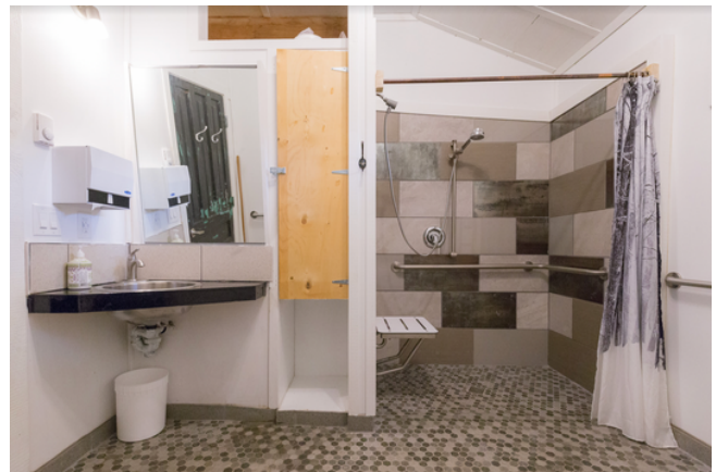
Barrier-free shower with bench and grab bars
